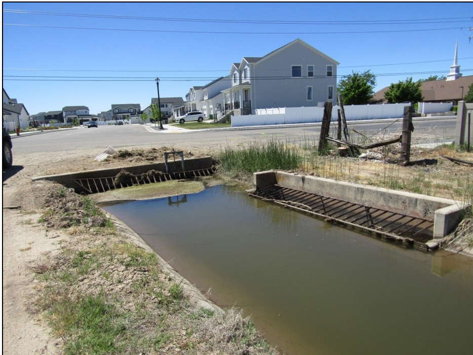
42DV158; Main canal at 300 North showing trash racks, diversions, and culvert; looking south
